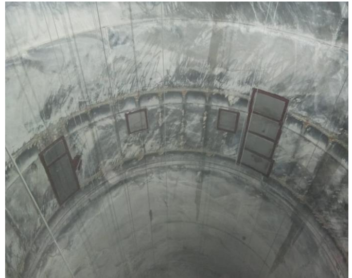
Protecting weld joint areas with Duromar EXP
