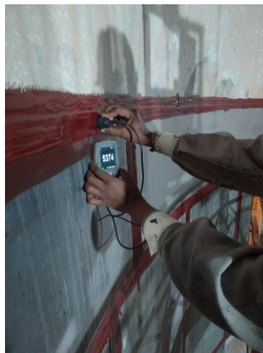
Protecting weld joint areas with Duromar EXP
