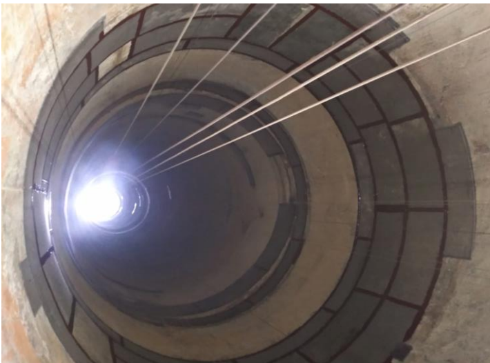
Rebuilding severely corroded portions of chimney stack with Duromar SAR and protecting corrosion sensitive areas with Duromar EXP.
