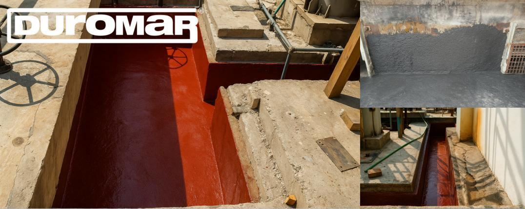
Repair & Rebuild of Acid Neutralisation Trench Lines using Duromar® DF-1301, DuroFil, and Duromar® DF-4301
