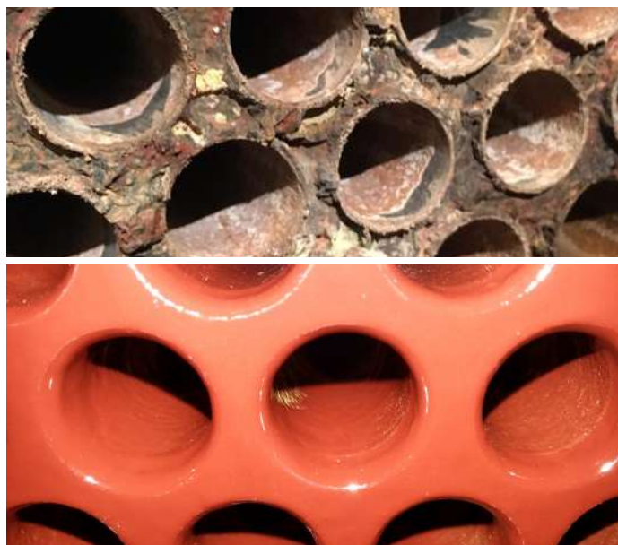
Heat-Exchanger tube inlets coated using plastocor Inlet System
