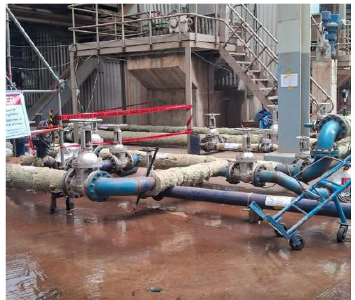
Boiler Tube Cleaning
