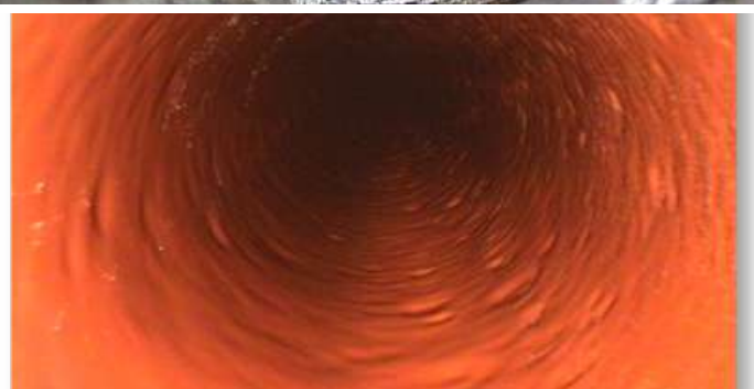
Heat Exchanger tubes upon application of plastocor® Tube Lining System
